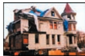
"Kurrajong" was moved 12 feet and placed on a new foundation.
